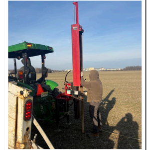
Snow fence posts being installed on CR 689 Cross Keys Bypass in Washington.
