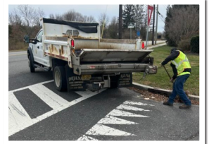
Inlet cleaning on CR 610 Clayton Road in Clayton.
