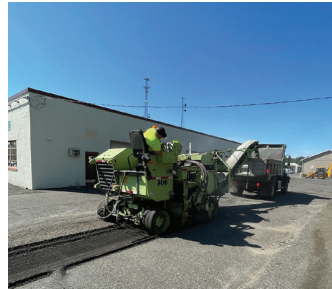
Milling in the Clayton ambulance parking yard for battery recharge area.
