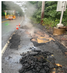
Cleanup and repair of damage to CR 651 Greentree Road in Washington Township caused by a high voltage electrical line which fell on and ignited the road.
