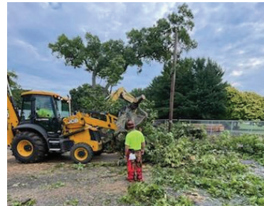
Removal of a very large tree from CR 689 Glassboro Cross Keys Road in Glassboro. In addition to a high degree of coordination and collaboration, this massive tree required a bucket truck, backhoe, and excavator to cut it up and clear it from the road.
