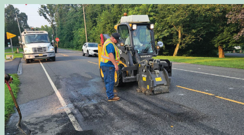
Joint repair on CR 553 ALT in Mantua. The asphalt over the existing concrete roadway was raised and needed to be milled off to remove the bump in the road.
