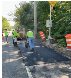
Cleanup and repair of damage to CR 651 Greentree Road in Washington Township caused by a high voltage electrical line which fell on and ignited the road.
