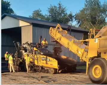
Recent upgrades at the Fire Academy's new burn building include paving the surrounding area and the installation of a new storm pipe behind the building to assist with water runoff during training activities
