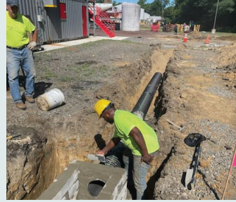
Recent upgrades at the Fire Academy's new burn building include paving the surrounding area and the installation of a new storm pipe behind the building to assist with water runoff during training activities
