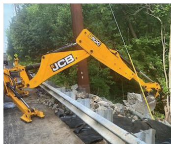
Crews perform washout repair on Kings Highway east of Wolfert Station Road in East Greenwich. Approximately 10 loads of fill dirt were placed in this very large washout. The area was then covered in fabric to help control future erosion and, finally, four truckloads of riprap rock was installed to finish the repair.
