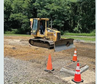
Recent upgrades at the Fire Academy's new burn building include paving the surrounding area and the installation of a new storm pipe behind the building to assist with water runoff during training activities
