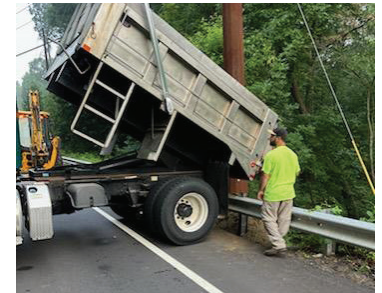
Crews perform washout repair on Kings Highway east of Wolfert Station Road in East Greenwich. Approximately 10 loads of fill dirt were placed in this very large washout. The area was then covered in fabric to help control future erosion and, finally, four truckloads of riprap rock was installed to finish the repair.
