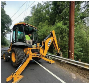
Crews perform washout repair on Kings Highway east of Wolfert Station Road in East Greenwich. Approximately 10 loads of fill dirt were placed in this very large washout. The area was then covered in fabric to help control future erosion and, finally, four truckloads of riprap rock was installed to finish the repair.
