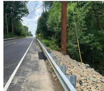
Crews perform washout repair on Kings Highway east of Wolfert Station Road in East Greenwich. Approximately 10 loads of fill dirt were placed in this very large washout. The area was then covered in fabric to help control future erosion and, finally, four truckloads of riprap rock was installed to finish the repair.
