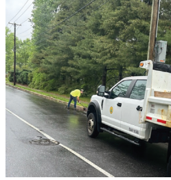
Inlet cleaning on CR 634 Fish Pond Road in Washington Township.
