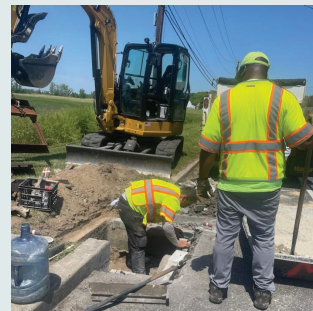
Repairs to replace broken inlet frame and casting on CR 662 High Hill Road in Logan.
