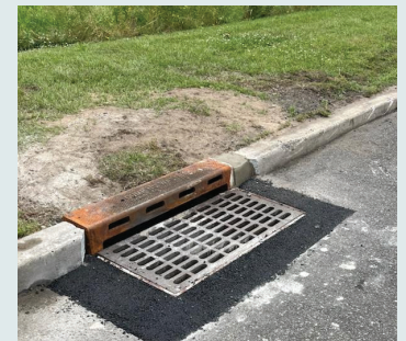
Repairs to replace broken inlet frame and casting on CR 662 High Hill Road in Logan.
