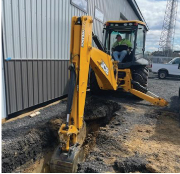
Drainage system being installed in front of the new Fire Academy building in East Greenwich
