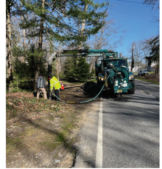
Vacuum truck cleaning inlets and storm pipes on CR 667 Aura Road in Elk Township
