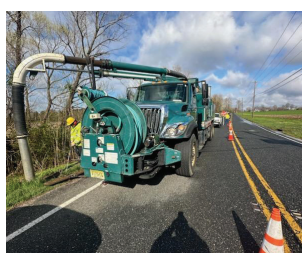
Vacuum truck cleaning inlets and storm pipe on CR 648 Ogden Station Road in West Deptford
