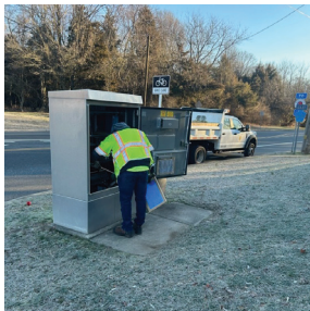
Maintenance on traffic signal control cabinet at CR 610 East Academy Street and CR 655 Fries
