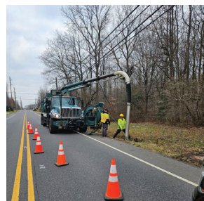
Vacuum truck cleaning of a clogged storm pipe on CR 680 Harmony Road in Greenwich
