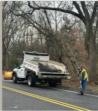
Patch truck at work on CR 667 Cedar Road in Harrison Township; pothole patrol on CR 678 Mount Royal Road in Mantua Township
