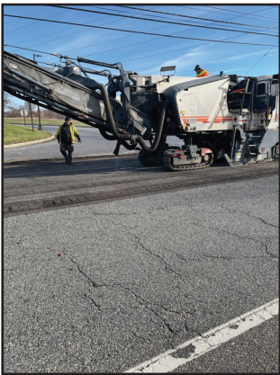
South State Crew milling CR 643 Grove Road in West Deptford in preparation of paving.
