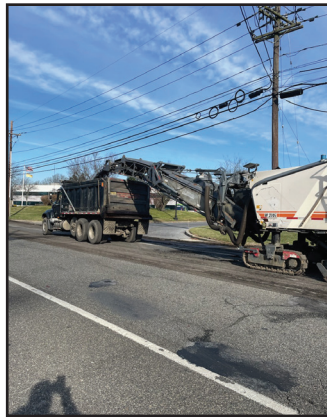
South State Crew milling CR 643 Grove Road in West Deptford in preparation of paving.
