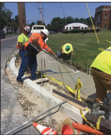
Accessible sidewalk ramps installation at the intersection of Red Bank Avenue and Evergreen Avenue in Woodbury
